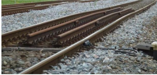
Figure 3. Transition zone with a large differential settlement.
