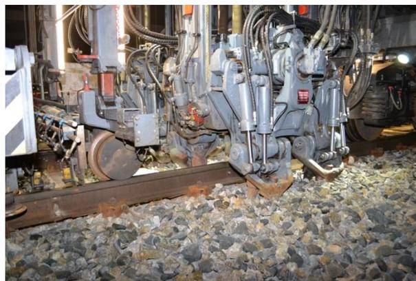
Figure 7. Tamping in a transition zone.
