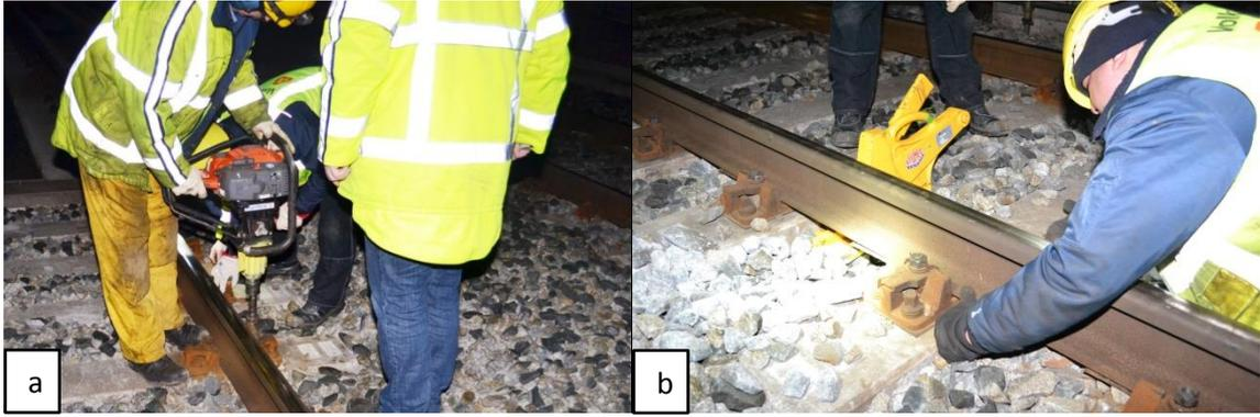
Figure 8. Adjustment of the fasteners.
