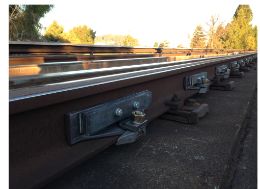
Tuned Dampers on ballastless track
