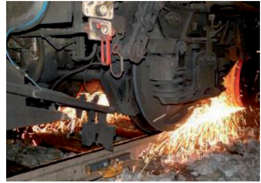
Rail grinding
