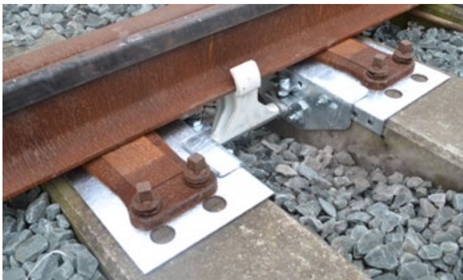
Figure 10: DeltaSwitch pendulum block under the switch rail of a 1: 9 switch without stiffener
