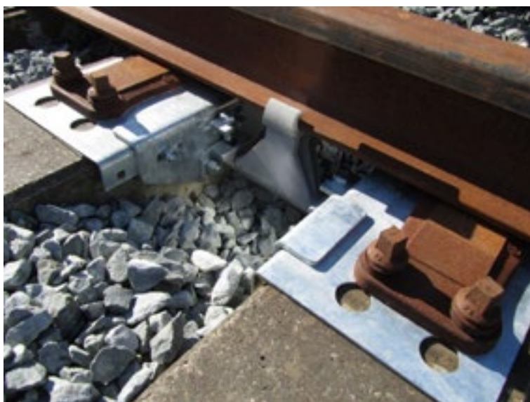
Figure 5: Overview of a built-in DeltaSwitch frame with pendulum
