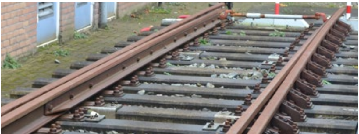
Figure 9: Switch with L-shaped stiffener on the switch rail (switch panel without DeltaSwitch)
